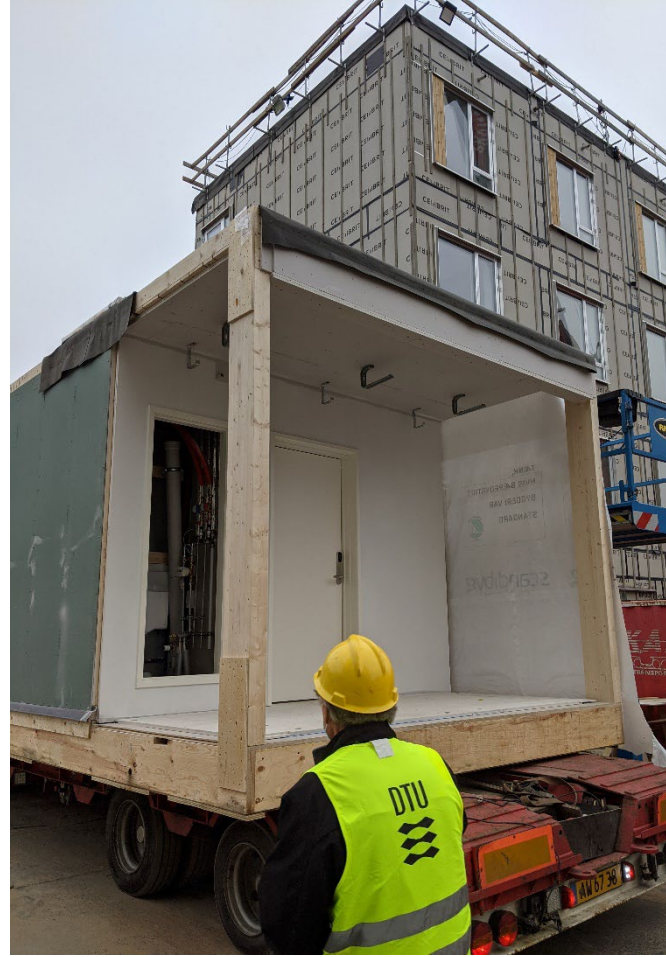
Includes the hallway and mechanical cabinet
